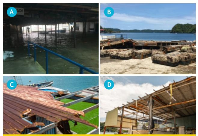
Figure 1: Sam's Tours super storm Surigae damage; a) inside the dive shop; b) dock floats; c) roof damage; d) building damage; 2021, photos by Sam Scott
